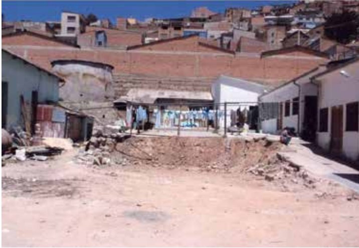
Figure 4 – Construction of the Burn Unit, Oruro, Bolivia
