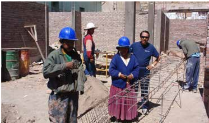
Figure 5 – Construction of the Burn Unit, Oruro, Bolivia
