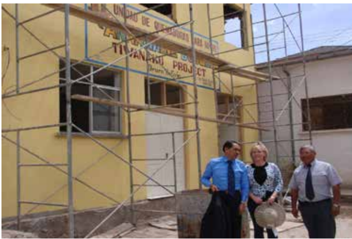
Figure 6 – Construction of the Burn Unit, Oruro, Bolivia
